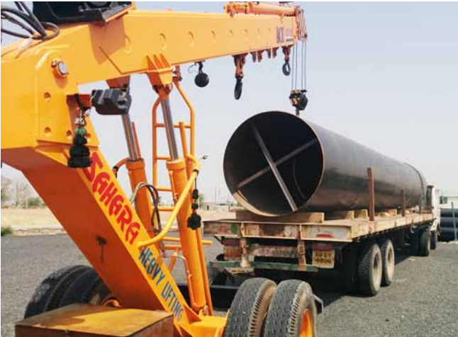
Figure B.2.3 Unloading of 1800 mm diameter pipe at storage yard
